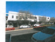
VIEW OF SOHO ON SUMMER
