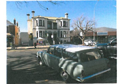
VIEW OF FINANCIAL SERVICES AND ADJOINING OFFICE BLOCK
