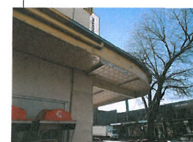
VIEW OF POST OFFICE LANE AWNING AND SIGNAGE
