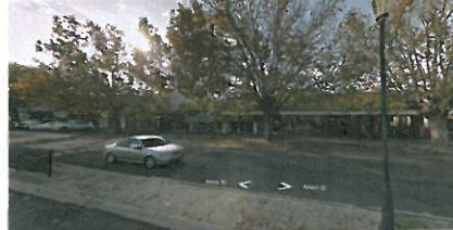
VIEW OF BUILDINGS TO BE DEMOLISHED
